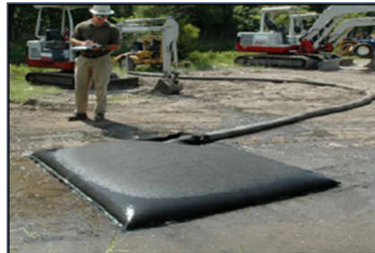
Plate 3-2 Silt Bag under inspection
