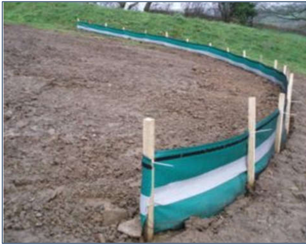
Plate 3-4 Embedded Silt Fence
