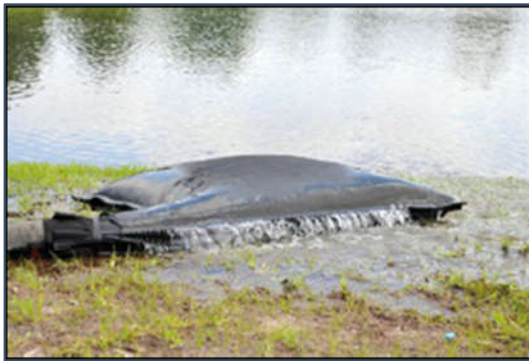
Plate 3-1 Silt Bag with water being pumped through.
